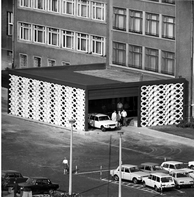
Figure 3. Hidden entrance in the Stasi building 13
